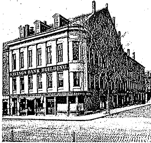
East Boston Savings Bank Building.
