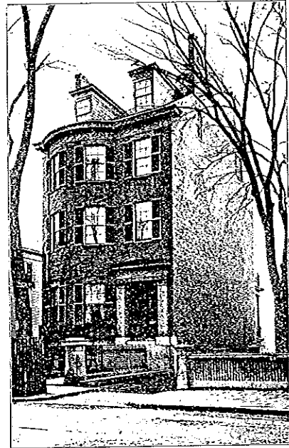
Residence Hon. John H. Sullivan, Webster Street.
